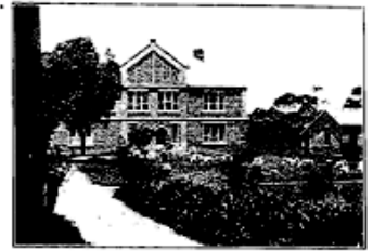
EDWARDS INDUSTRIAL HALL Cost of electric lighting, fixtures, wiring, labor, share of power line, $1,100.00
