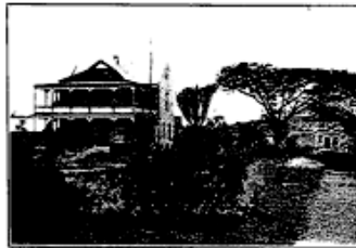
STANWOOD COTTAGE, TEACHERS' HOUSE Cost of electric lighting, fixtures, wiring, labor, share of power line, $550.00
