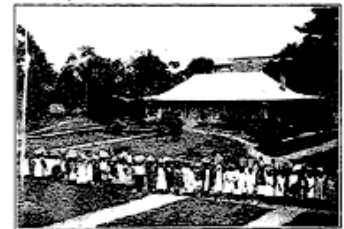
MISSION HOUSE, TEACHERS' AND VISITORS' ROOMS Cost of electric lighting, fixtures, wiring, labor, share of power line, $150.00
